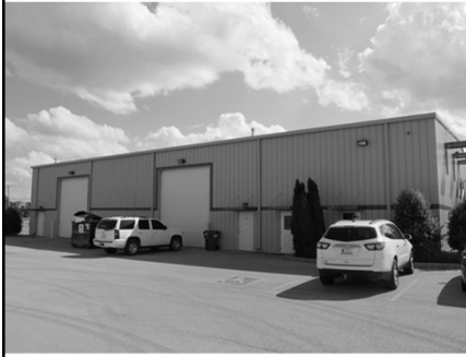
Guthrie Fire Station
